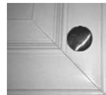
Representative of acceptable miter joint
